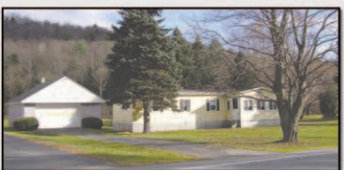
Near Quaint Village $69,900 Nice mobile home with over an acre of land, huge yard, and large detached 2-car garage. Offering 2 nice bedrooms, 1 bathroom, an enclosed porch, and lovely deck in the back for those summer barbeques. Just outside the village, close to dining, shopping and more! #18588
