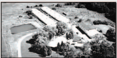
Multi-Use Commercial/Industrial $1,180,000 Beautiful bluestone ranch with attached garage (needs some updating), two large warehouse buildings, plus an additional office building with warehouse space, garage bays and 4+ apartments above. All on 10+ acres with paved parking, pond and with more available! #19376
